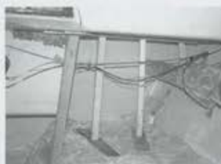
Brace are positioned to hold the new glass in place. Add shims to the bottom to adjust to the proper height.
